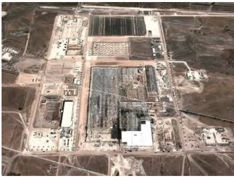
HONDA Celaya, Mexico Opened February 2014 Est. Production: 322K
